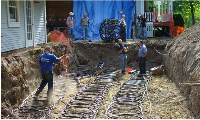
Installation of ground source heat system, courtesy of Sandra Cannon
