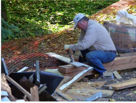
Nails pulled from siding and both materials reused, courtesy of Sandra Cannon
