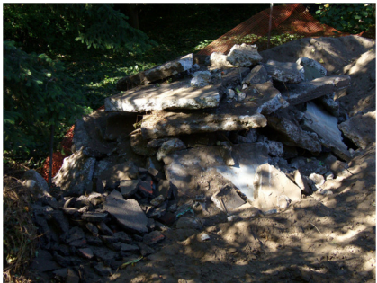
Concrete to be crushed and reused as fill for new patio, courtesy of Sandra Cannon
