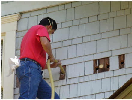
Installation of cellulose insulation, courtesy of Sandra Cannon
