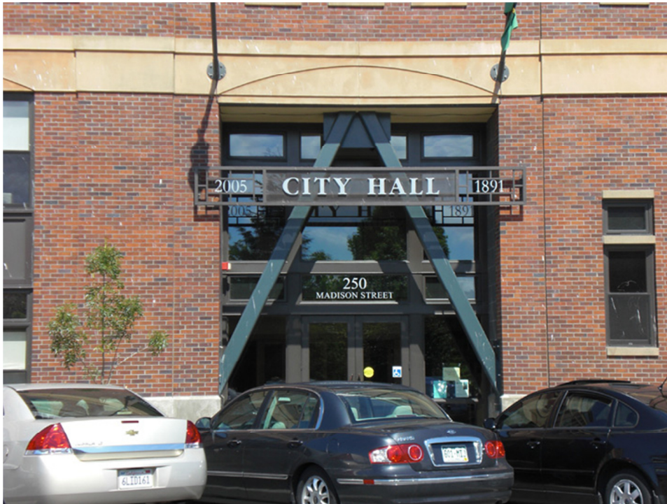
Seismic bracing at Annex entry ties to the historic structure, Kelly Laleman.
