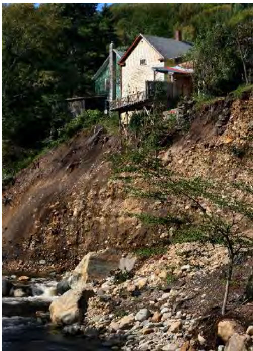
While landslides are a hazard of concern in Lake Arrowhead, property owners can use various strategies to reduce the risk. Photo source: Alex Drexel/FEMA
