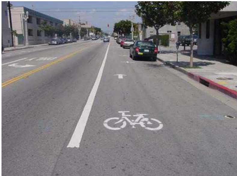
Figure 6.8 – Bike Lane Markings
