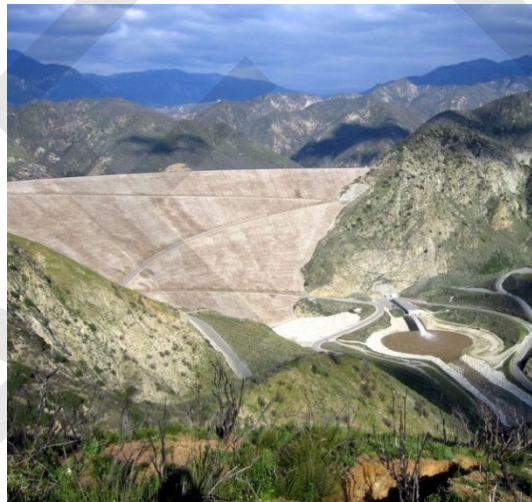
Seven Oaks Dam, Highland, California
