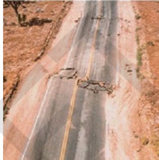
Surface fault rupture from the Landers Earthquake. Source: USGS Photo Gallery
