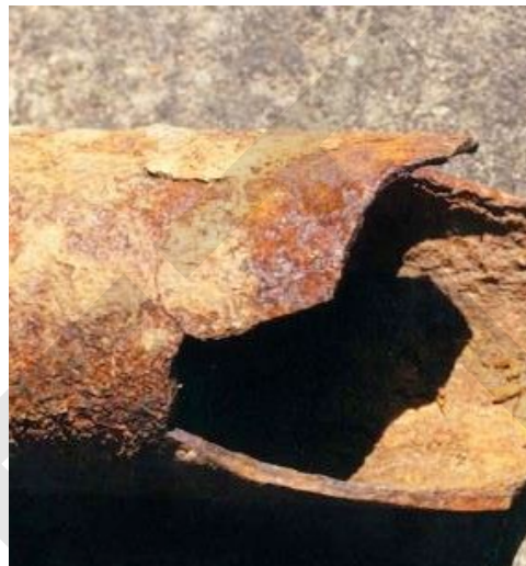
Corrosive soils can erode water main pipes, steel, and foundations, leading to hazardous conditions.
