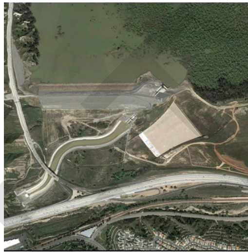
Prado Dam, California Source: USACE
