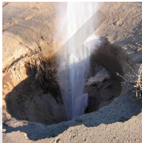
Photograph of pipeline rupture
