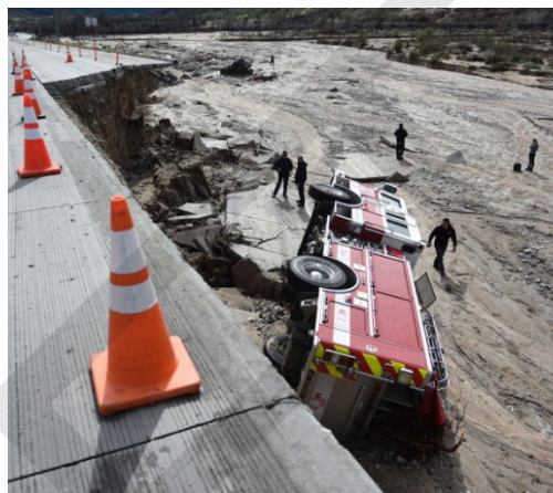
Flooding in 2017 along the Cajon Pass causes a freeway segment to collapse, taking with it a fire engine
