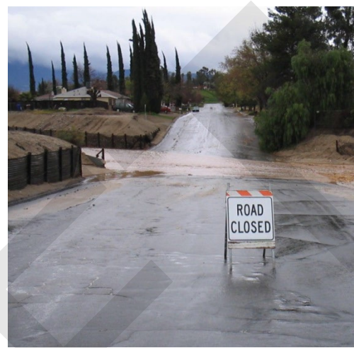
Flooding in suburban areas of San Bernardino County can block access to residential neighborhoods.
