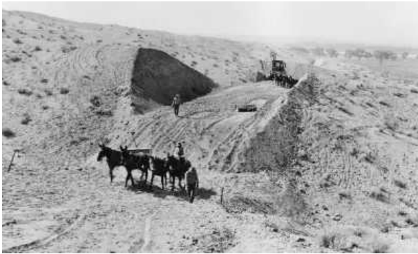
Photo source: California Department of Transportation 2016
