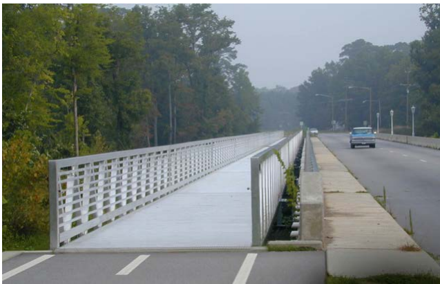
Retrofit of an aluminum bridge to an existing highway bridge with inadequate pedestrian facilities. This is typically a less expensive option than widening of an existing bridge. Photo source: MAADI Group
