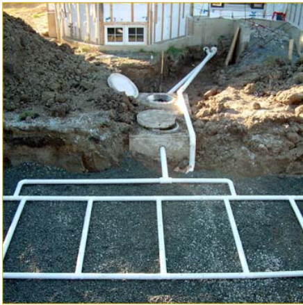
Underground setup of septic system.
