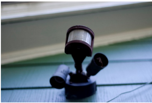
Property owners can connect their outdoor lights to motion detectors. These low-cost devices can help discourage crime by making it harder for lawbreakers to hide. Photo source: Joey Parsons.
